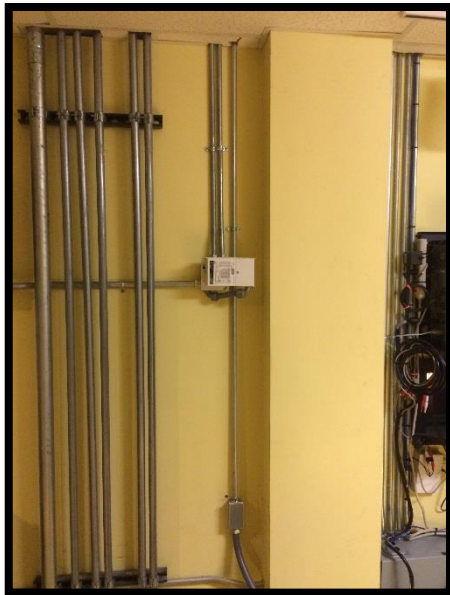
Electrical Conduit from the ceiling and connection to SLG rack
