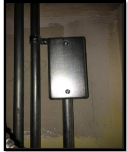
Wall Penetration (Auditorium side and Booth side- above ceiling) - JBox Cover (booth side)
