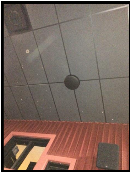
AP black cover mounted on the ceiling grid
