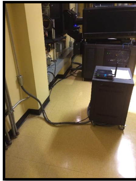
Electrical Conduit from the ceiling and connection to SLG rack
