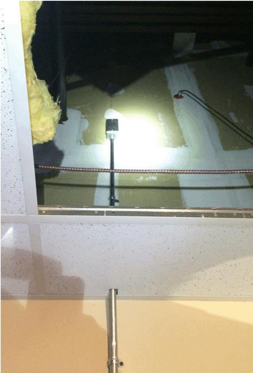
*image02* -upper handy box covering penetration and conduit
