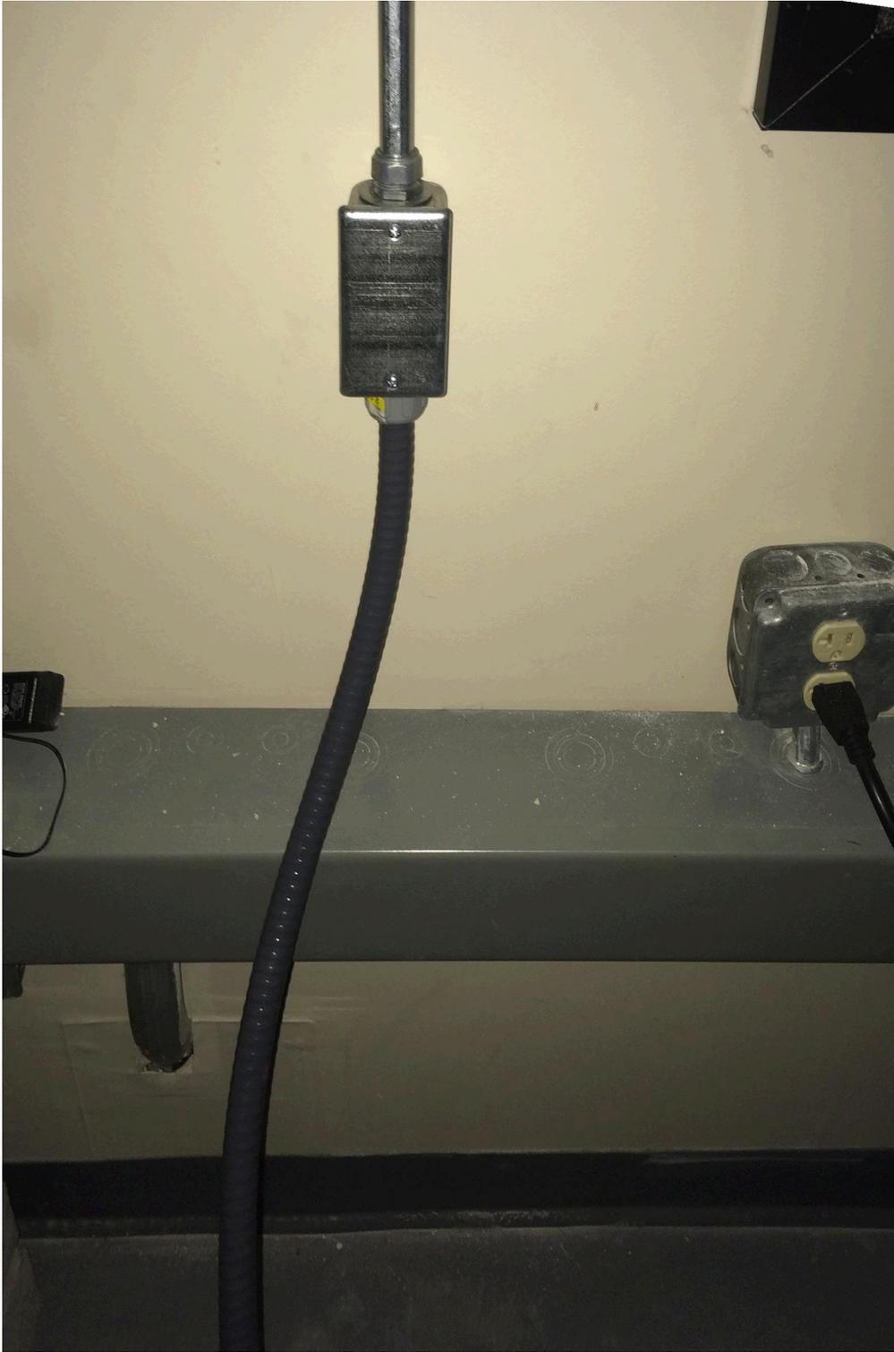
*image03* -lower handy box single gang with liquid tight from rack
