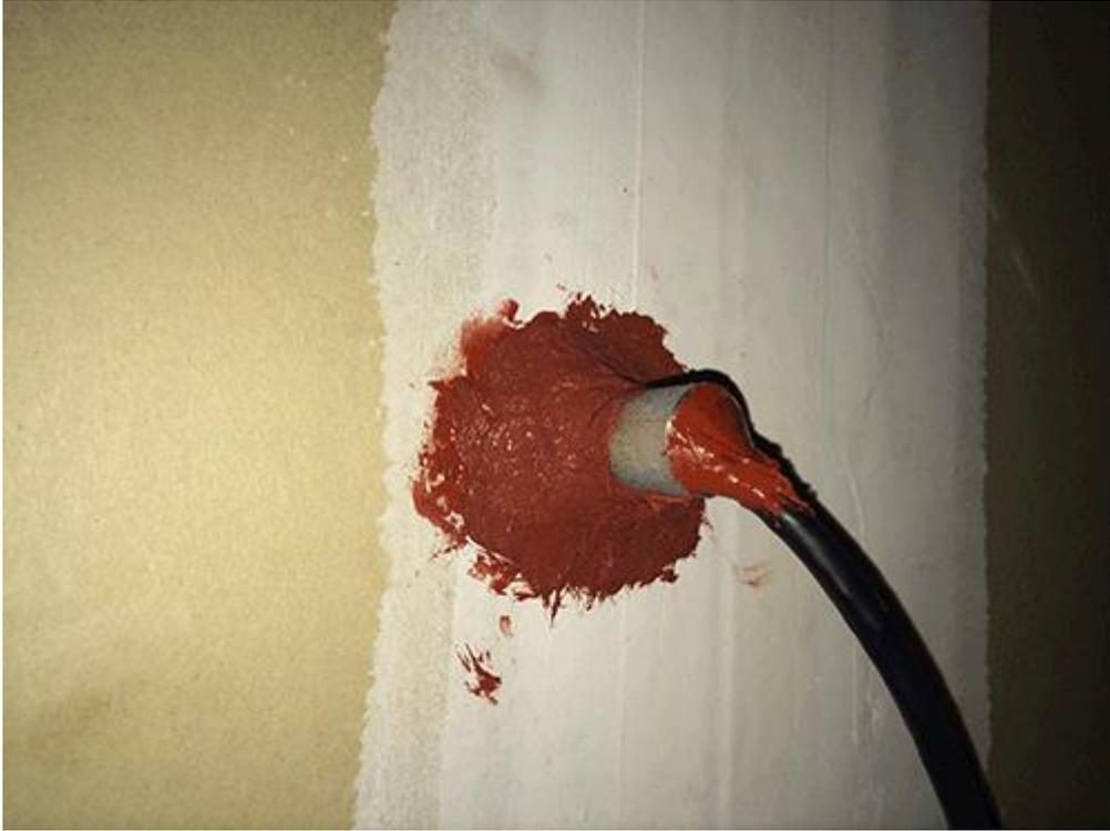
*image01* -drywall penetration and fire resistant filling
