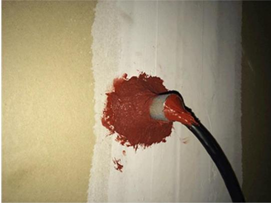
example of drywall penetration and fire resistant caulk
