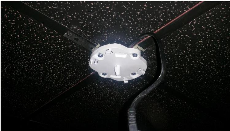
Plastic mount attached to metal clips with metal tab extended
